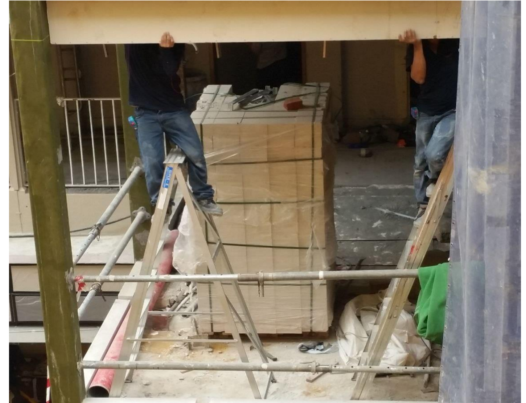
Above the guardrail next to the edge of the building
